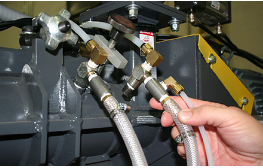
Air assisted jet assembly removed from the mixing chamber for physical calibration.
