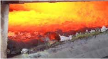
Exhibit A: 4-Month-Old Lining Stated: They Cleaned It Every Day.
