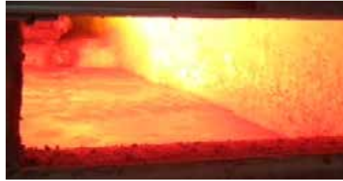
Exhibit B: Furnace Lining 3 Years Old Cleaned Properly
